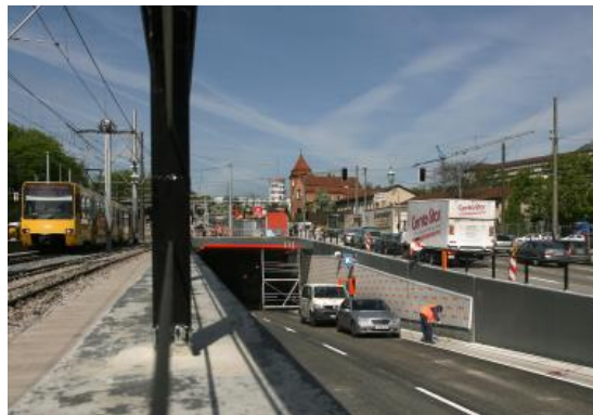
Figure 3: Slope after tunnel exit
